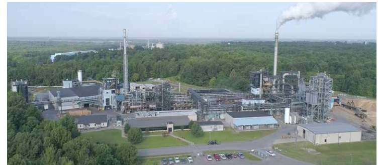
Ingevity's Wickliffe, Kentucky, plant manufactures activated carbon products used in automotive evaporative emissions systems, food, beverage and industrial purification applications.
